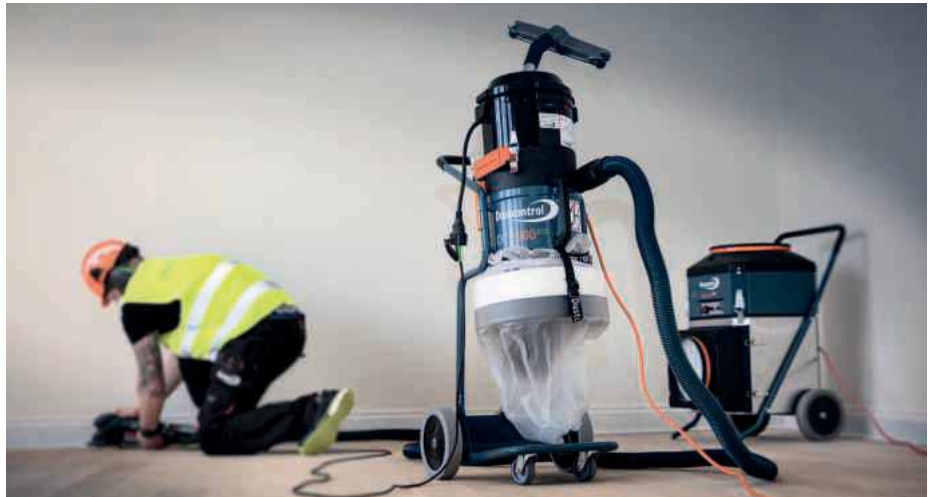
A worker using the DC 2900L and AirCube 1200
