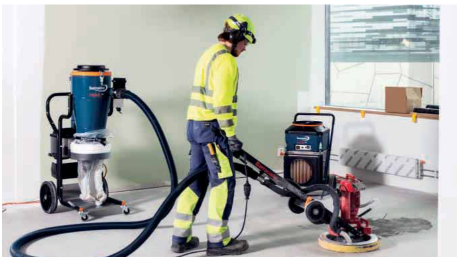
Floor grinding using the DC Tromb and AirCube 1200
