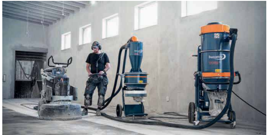
The DC Storm being used for floor grinding
