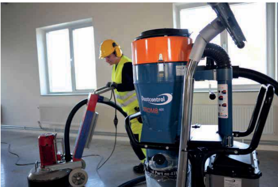
The DC Tromb being used in floor grinding
